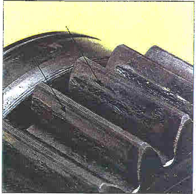
Pitting, scoring and galling can occur when the gear material endurance limit is exceeded. Lubrication problems can also contribute to these conditions.
